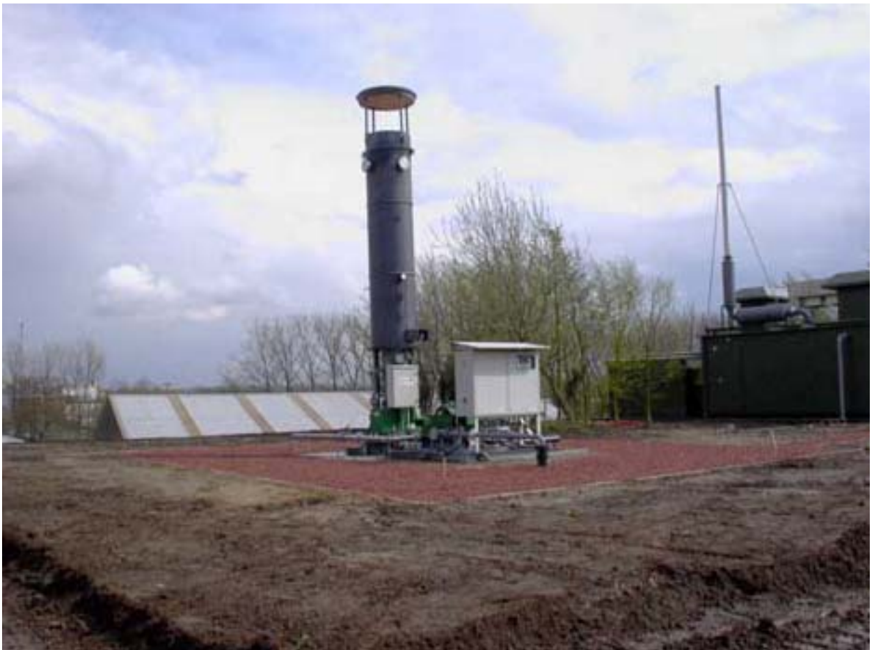
Typical biogas extraction unit.
